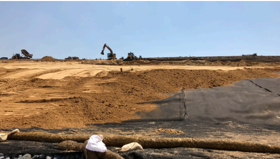
Ongoing capping of Freshkills’ West Mound, the last remaining landfill section to be capped at the site.
