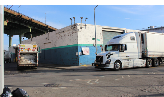
IESI Corporation Transfer Station, Court Street, Brooklyn, NY
