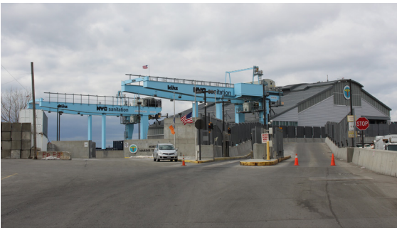
North Shore Marine Transfer Station, Flushing, NY
